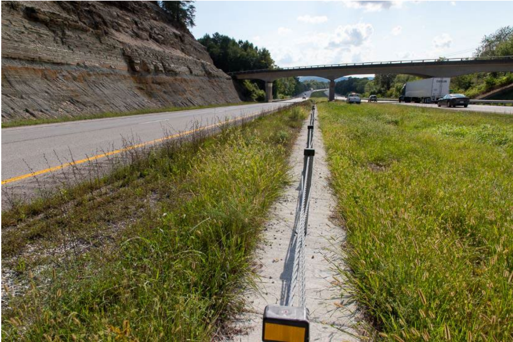
Figure 3: View of Plots in the Cable Barrier Trial on September 14, 2021 (110 Days After Treatment)
