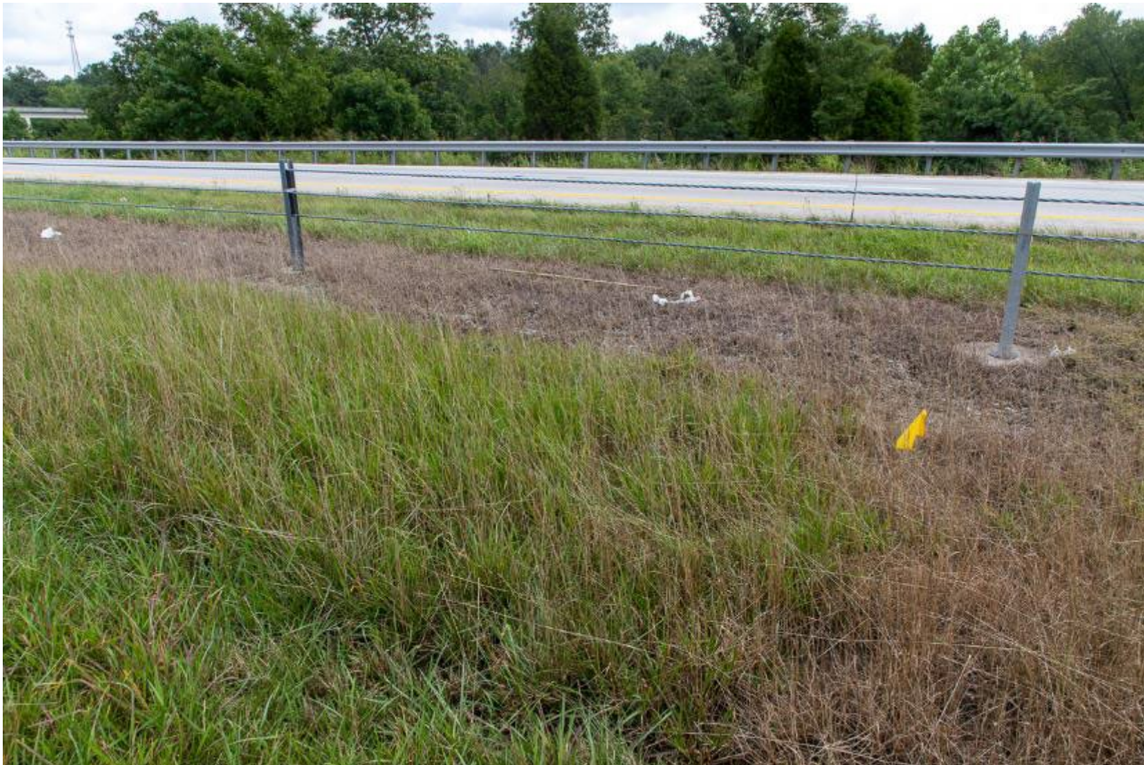
Figure 6: Perspective + Esplanade (Treatment 5) on August 4, 2020 (63 Days After Treatment) No grass damage beyond spray pattern.
