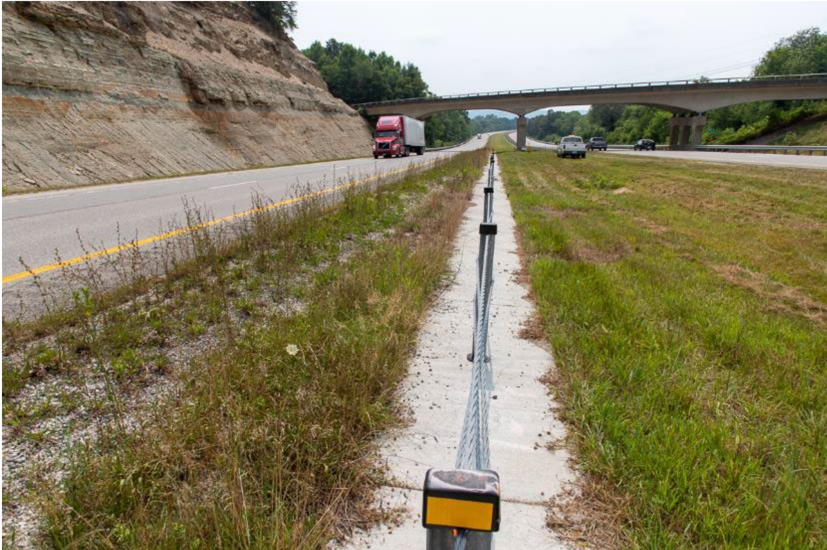
Figure 2: View of Plots in the Cable Barrier Trial on July 29, 2021 (63 Days After Treatment)
